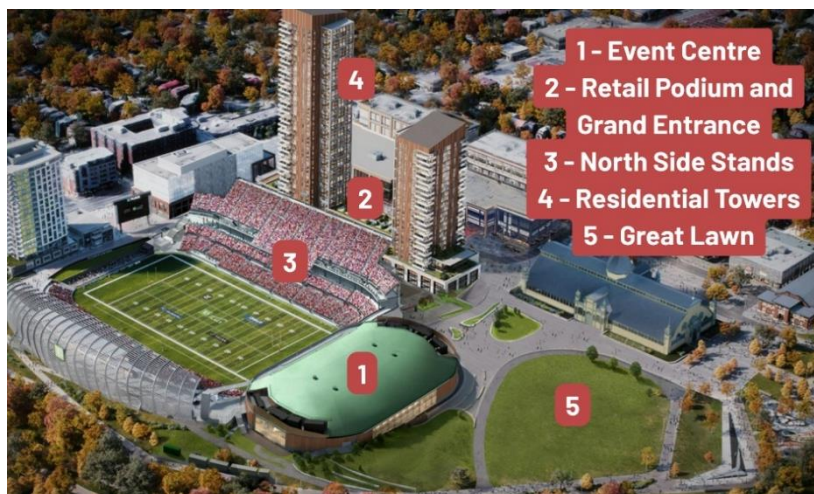
Lansdowne 2.0 Redevelopment (Photo Credit: City of Ottawa)
